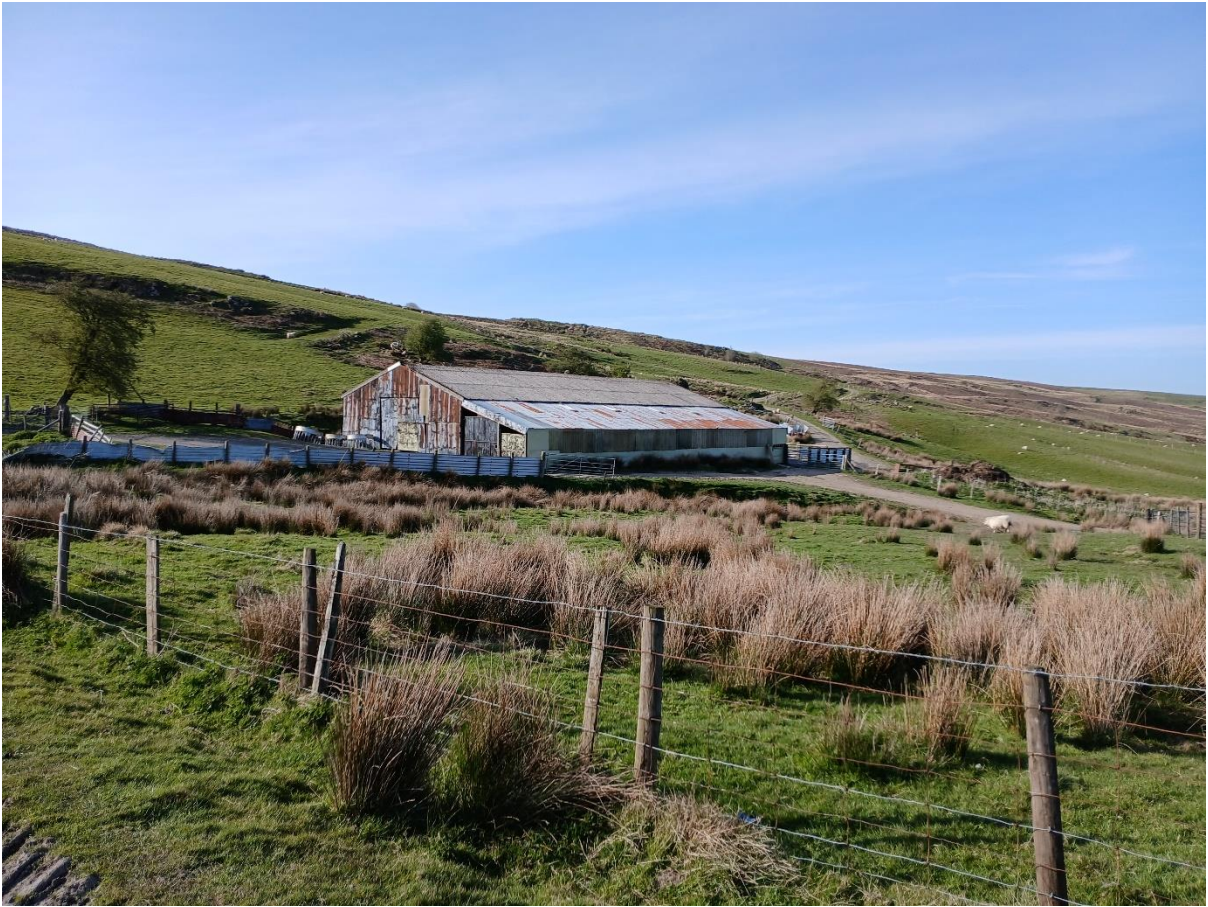
Photo 1: Onsite barn at Y Glonc used for sheep shearing etc in the north central area of the energy park site. Possible asbestos containing materials (ACMs) in building walls/roofing, but no tipped ACMs observed.
