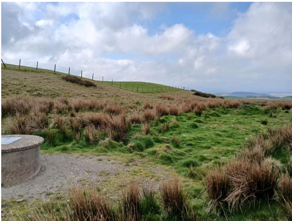
Photos 12 and 13: Unknown raised cylindrical feature – appears to be an access chamber, possibly related to a utility however this is unconfirmed – in southeast of site, near tipped material in photo 14 and 15.
